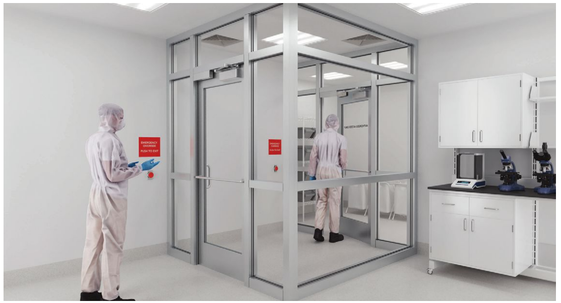
A new section has been approved for the 2027 I-Codes that will address interlocks, also known as control vestibules.
