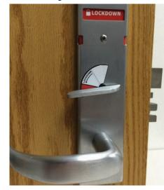
\*Auxiliary latch deadlocks latchbolt when door is closed. Inside lever is always free for immediate egress \*Interior cylinder operated indicator available in limited functions
