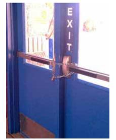
Fig. 1: Exit doors in a school, chained to provide security. This locking method does not meet IBC, IFC, or NFPA 101 requirements for free egress. (Photo: Wayne Ficklin, Architect)
