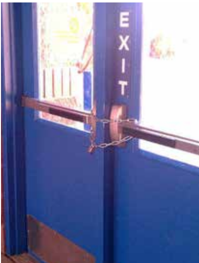
Fig. 1: Exit doors in a school, chained to provide security. This locking method does not meet IBC, IFC, or NFPA 101 requirements for free egress. (Photo: Wayne Ficklin, Architect)
