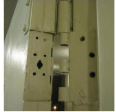
Constant latching flush bolts have an automatic flush bolt on the bottom, and the top is a spring-loaded bolt which is retracted manually to open the door. These bolts provide a higher degree of security than the other two because the inactive leaf is more likely to be closed and latched properly. They can be an egress issue for some doors because the top bolt has to be retracted manually, and it is not within the accessible reach range. A coordinator is also required for this application.
