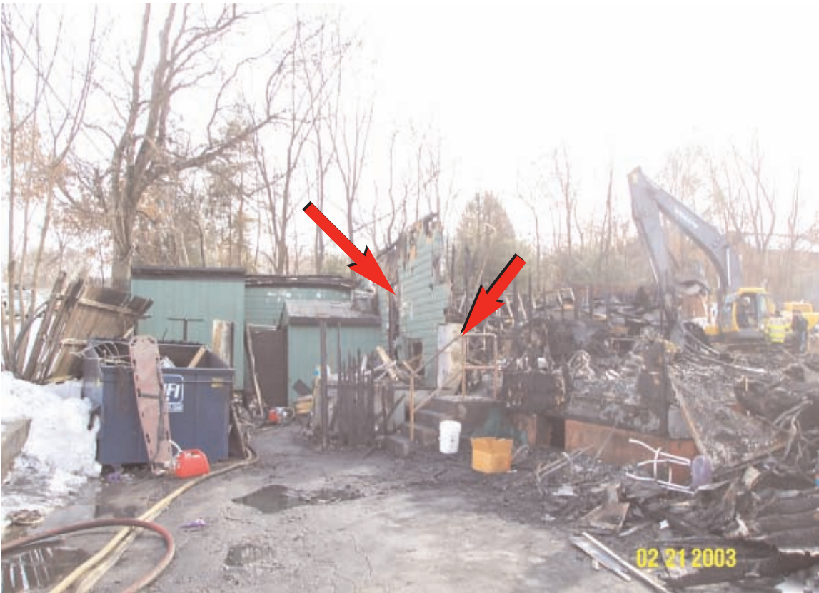
FIGURE 10 Exterior View Showing Both the Bar and the Kitchen Exits (see arrows) (NFPA).
