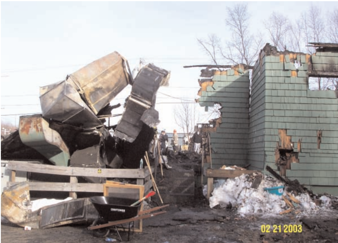
FIGURE 8 Exterior View of Exit Adjacent to Platform Area (NFPA).
