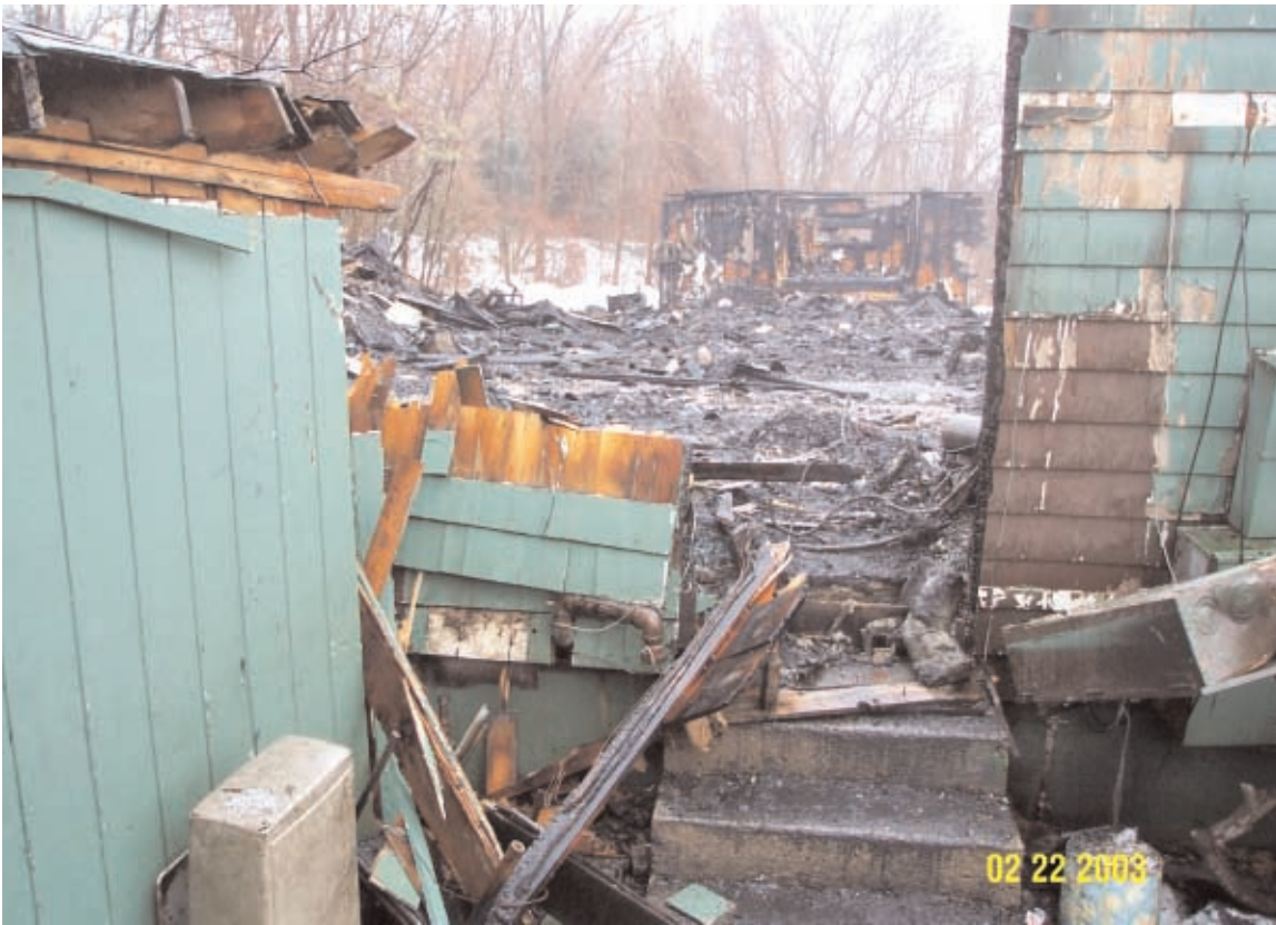
FIGURE 9 Exterior View Showing the Kitchen Exit Looking Toward the Platform Area (NFPA).
