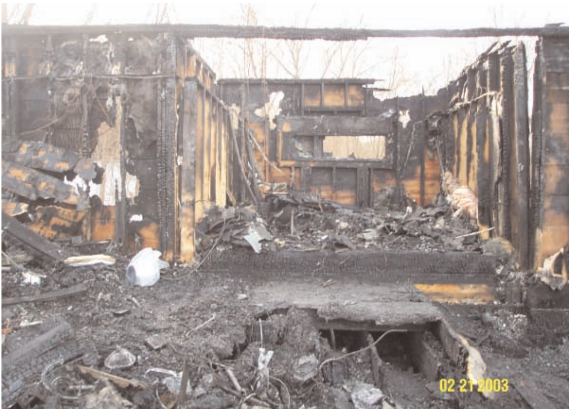
FIGURE 7 View from Interior of Club Showing the Platform and Drummer's Alcove (NFPA).
