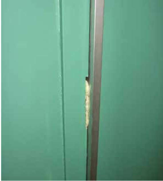
Using foam insulation to fill an existing hinge prep on a fire door assembly is not a method that is allowed by the manufacturers' listings.
