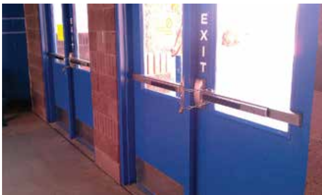
Exit doors in a school, chained to provide security. This locking method does not meet IBC, IFC, or NFPA 101 requirements for egress.
