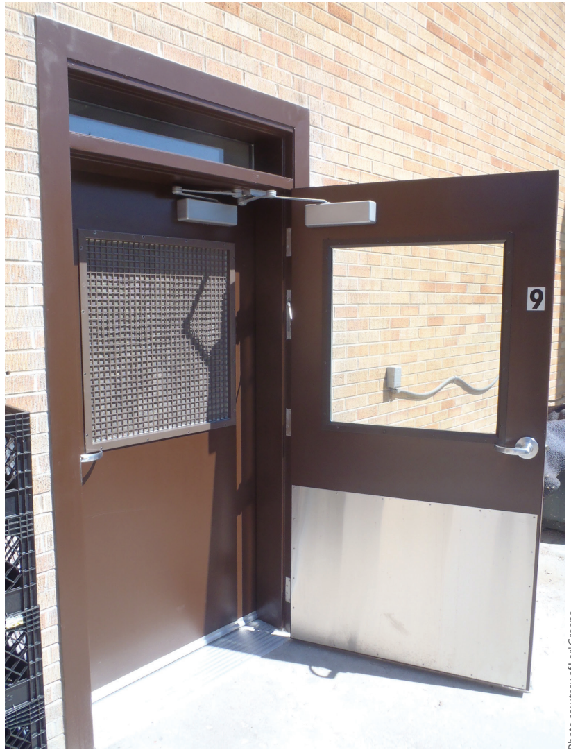
Two doors installed in the same frame do not meet the accessibility requirements for doors in a series, and may create a non-compliant egress situation.
