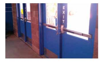
Exit doors in a school, chained to provide security. This locking method does not meet IBC, IFC, or NFPA 101 requirements for egress. Photo: Wayne Ficklin, Architect
