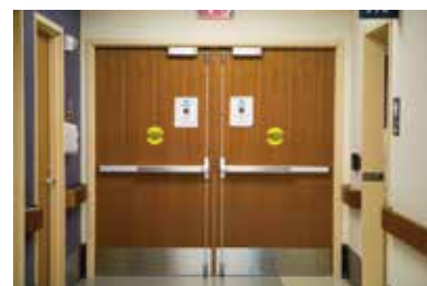
Controlled egress locks are allowed in some health care units, but staff must be prepared to facilitate egress if needed.
