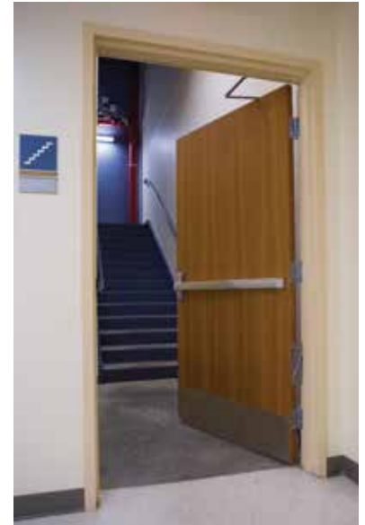
The stairwell reentry requirements vary between the IBC and NFPA 101; the IBC requires all stair doors to allow reentry with the exception of the discharge door.
