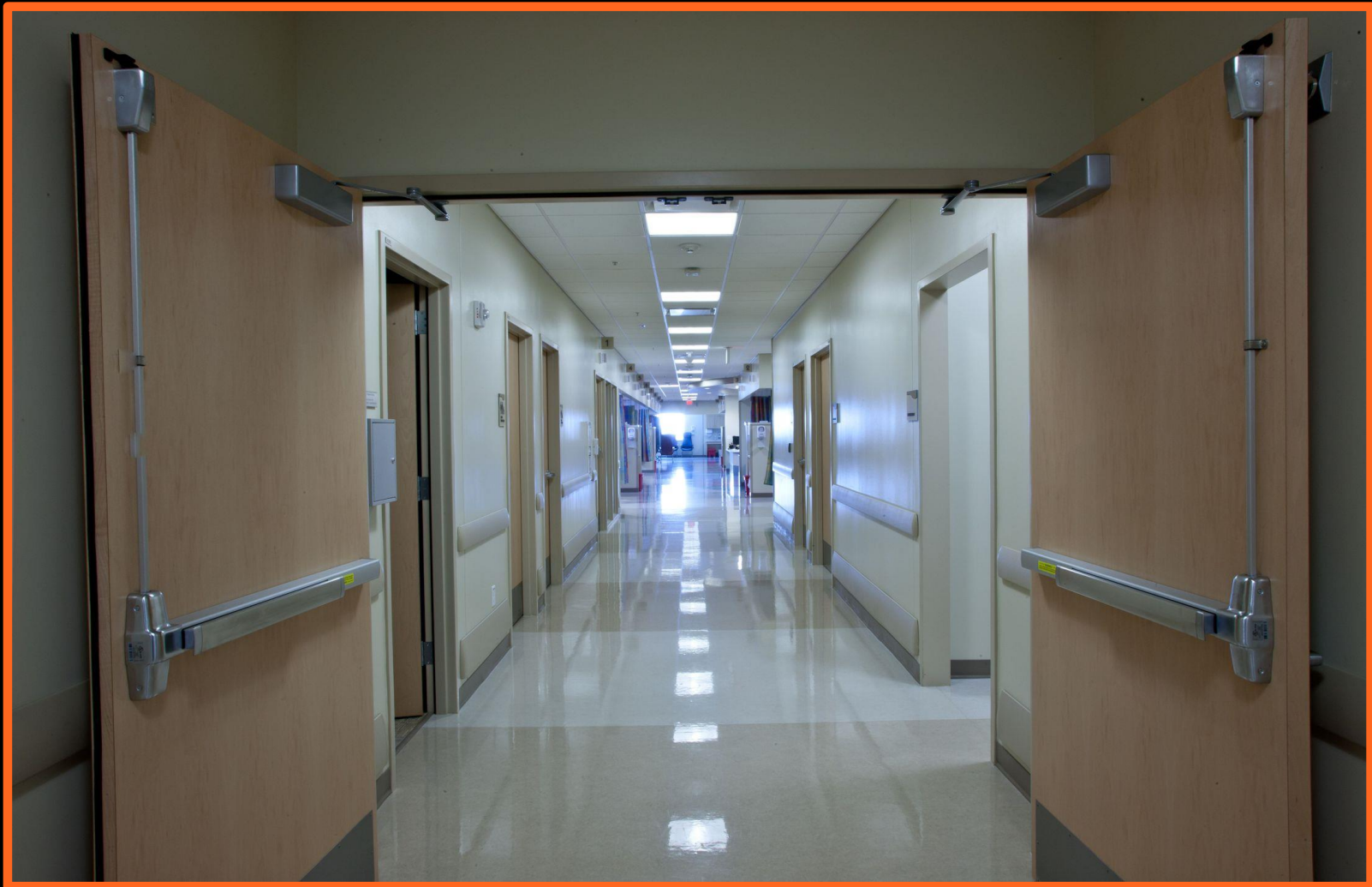
Swinging Doors with Builders Hardware
