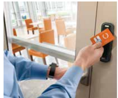
When a door equipped with an access control reader allows free egress using normal operation of the hardware, it is not typically considered one of the special locking arrangements.
