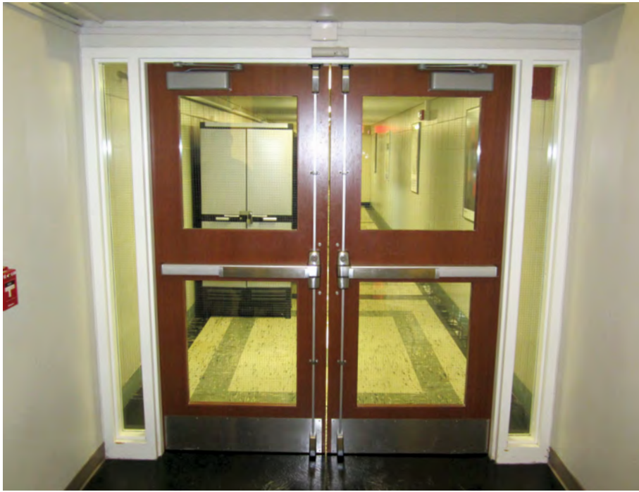
These doors were installed within the last six months and contain traditional wired glass, even though the doors are not fire-rated and the code requires impact-resistant glass in all doors.
